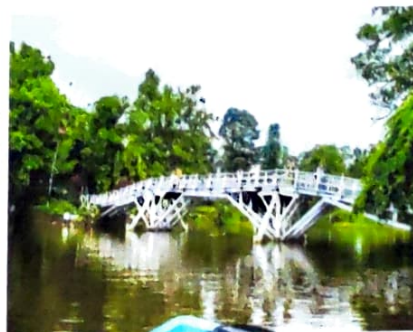
WARD'S LAKE BRIDGE
